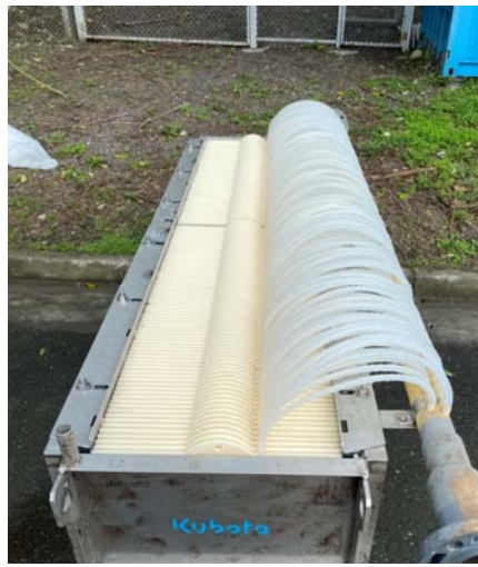
Ecologix PVDF element insert to Kubota module
