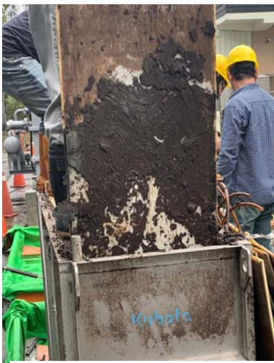
Kubota #510 element sludge caking
